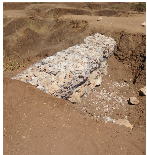
A completed gabion
