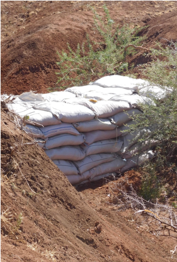
A completed soil bund
