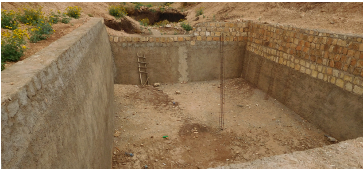
A birkad under construction
