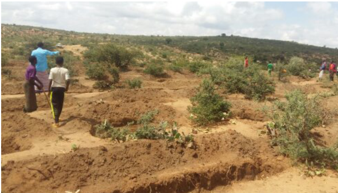
Community members digging trenches
