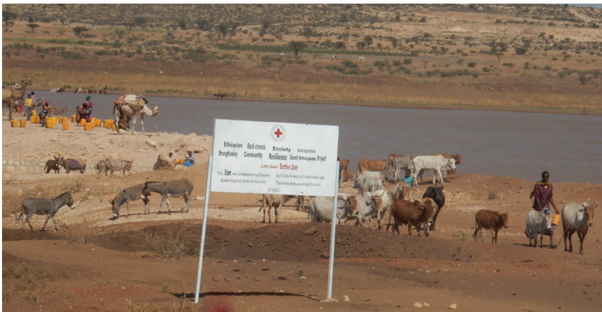
Laftagalol earthen dam
