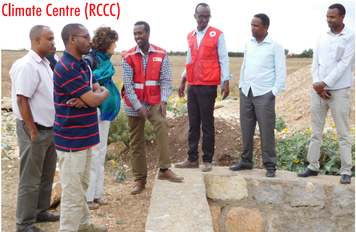
Staff of NLRC, ERCS and Wetlands International inspecting one of the birkads under construction
